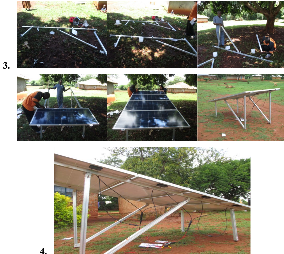
Figure 1. Mounting of aluminium profiles for 4 solar panels
