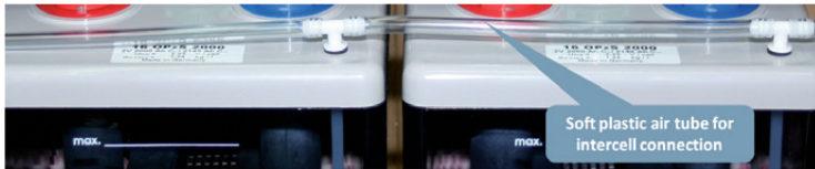
Figure 10: Connection between air tubes - I
