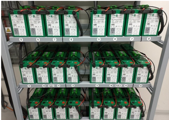
Figure 6.6.5-1 - Use of series and step connectors
